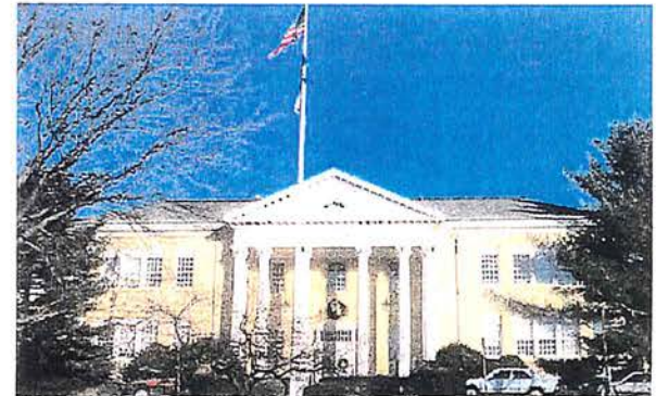
Town Hall situated along Myrtle Avenue fronting Avery Commons.
