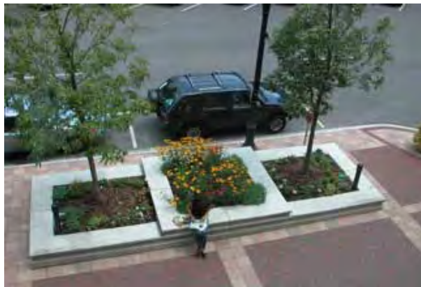
Trees in concrete planters (cast-in-place)
