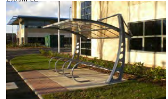
Figure 99: A bicycle parking shelter
