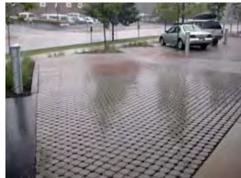
Pervious paving after a rain storm
