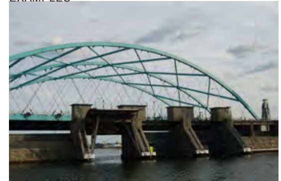
Figure 119: Floodgates in Providence, RI
