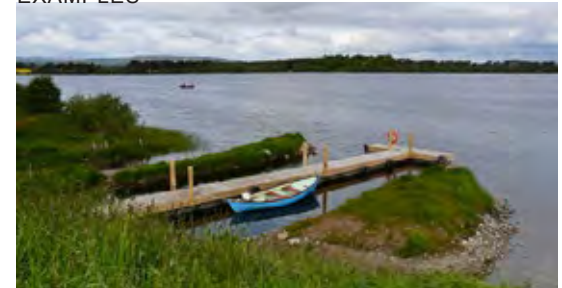
Figure 59: An example of a small dock
