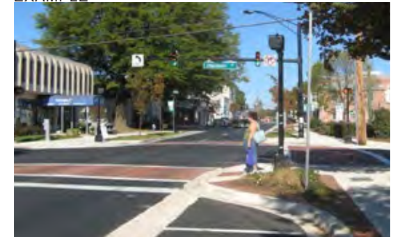
Figure 69: A curb extension reduces crossing distance
