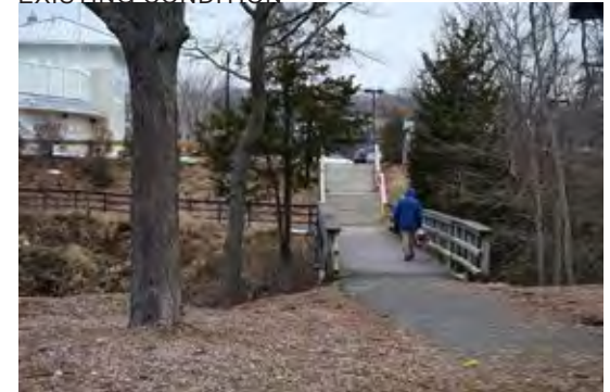
Figure 82: The pedestrian bridge that currently connects Levitt Pavilion and the Library with the Imperial Avenue Lot
