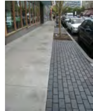
Porous pavers on a sidewalk
