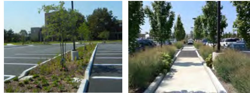
A bioswale in a parking lot | A walkway in a parking lot, lined by rain gardens
