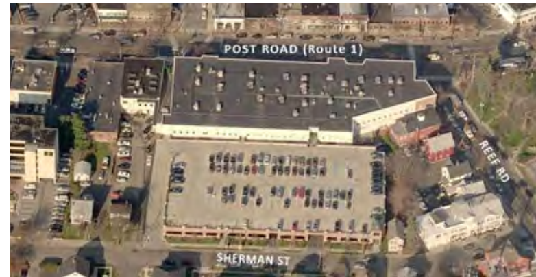
Figure 151: Example of a parking deck
