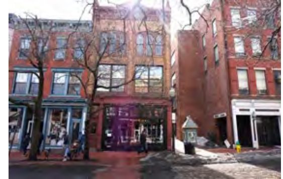
Figure 112: A parking deck is located behind buildings along Washington Street in SONO in Norwalk, CT, with access provided through a pedestrian passageway
